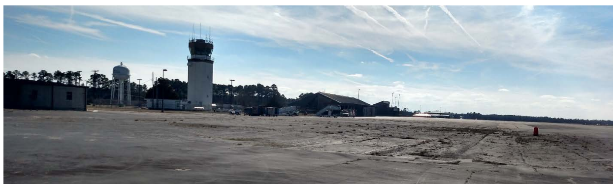
Figure 19: Taxiway, air control tower, and terminal building at runway.
