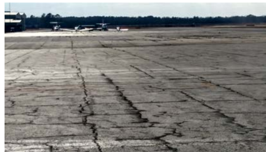
Figure G-3: Airfield pavement condition
